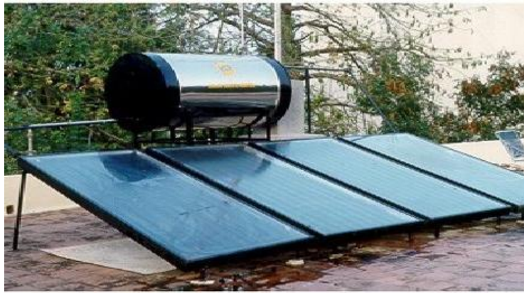
Figura 3. Colector solar de placas planas (China Suppliers, 2012).
